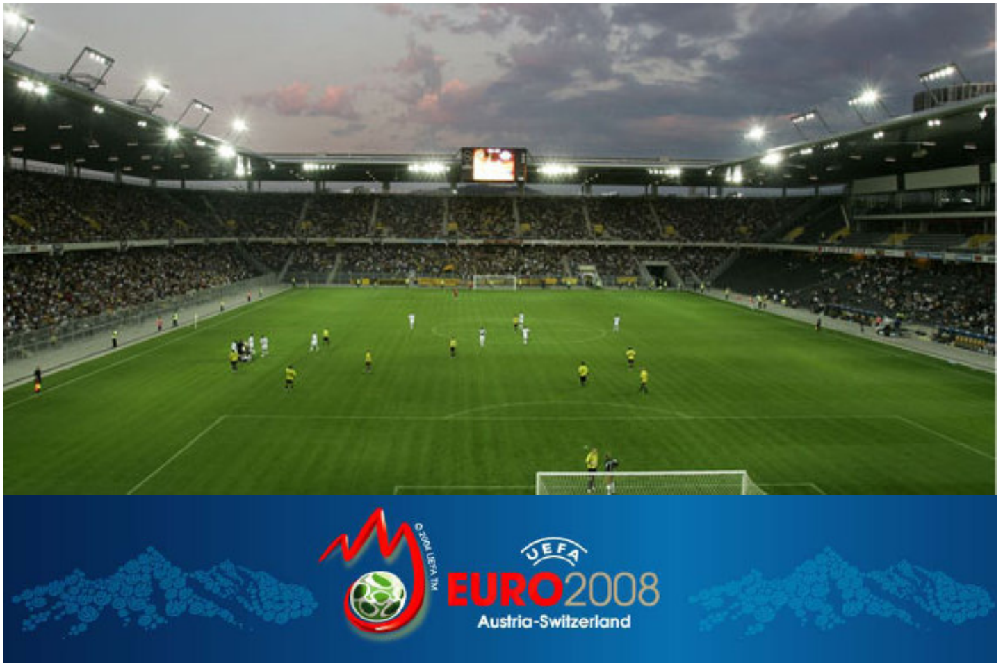
Above and below photos are Salzburg Wals-Seizenheim Stadium with Lexan* Thermoclear Sheet roofing
